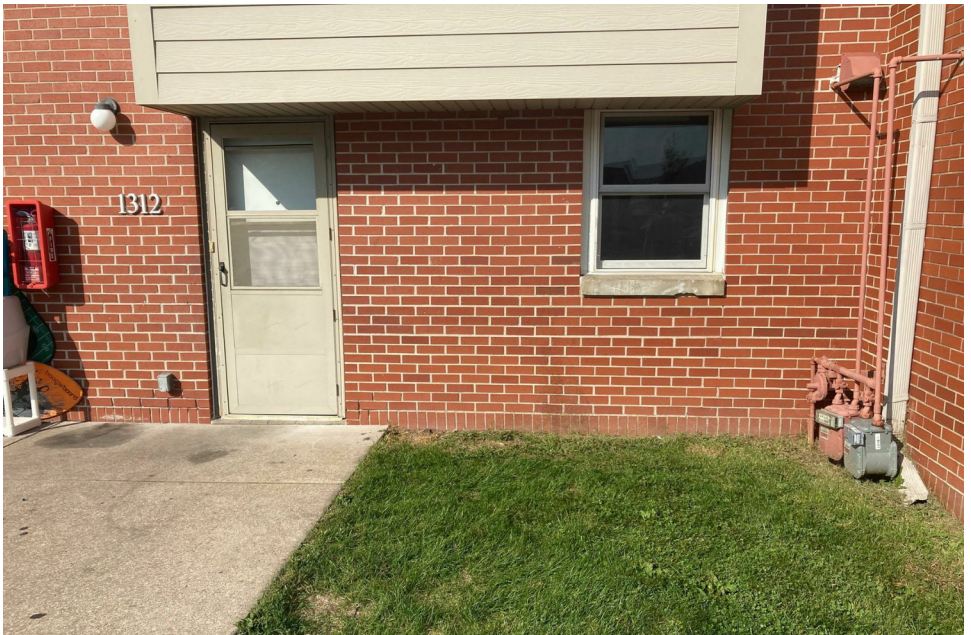
SOFFIT AT FIRST FLOOR WINDOWS
